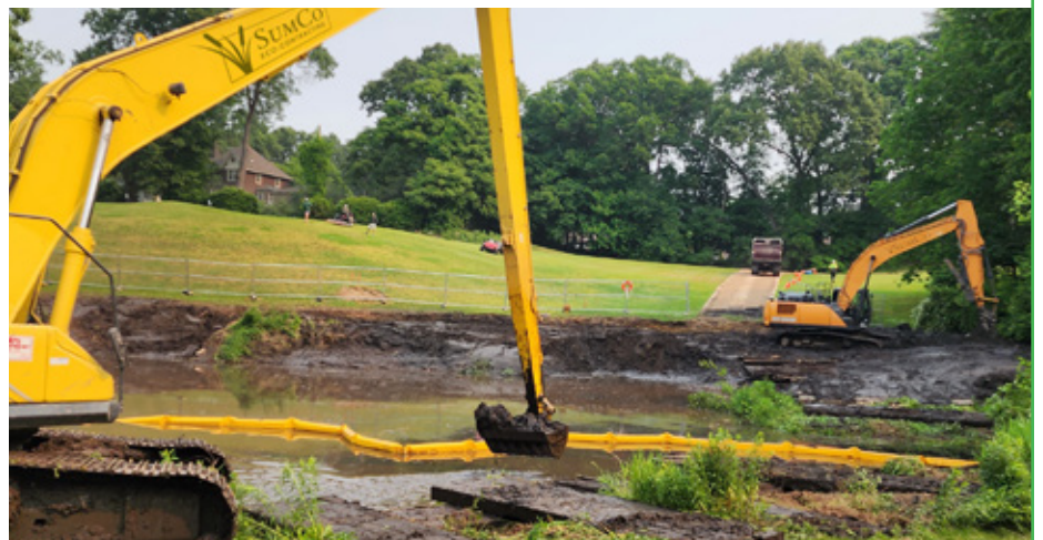
Completed in Spring 2023: Franconia Golf Course pond maintenance dredging, Springfield, MA
